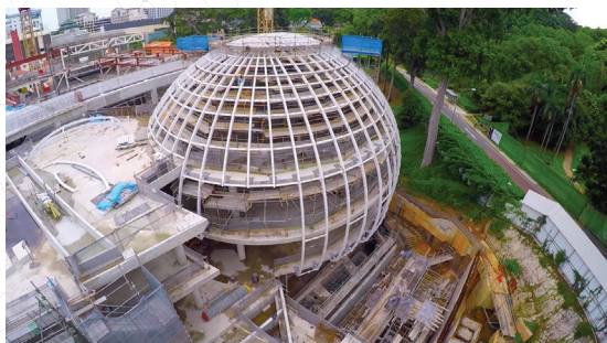
Putting the dome's structure together during construction of the Kwa Geok Choo Law Library
